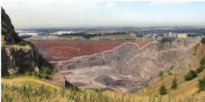
Fig. 3. Current (active) Bardon Hill Quarry, showing deep channels in the Precambrian bedrock resource filled with the Mercia Mudstone Group
